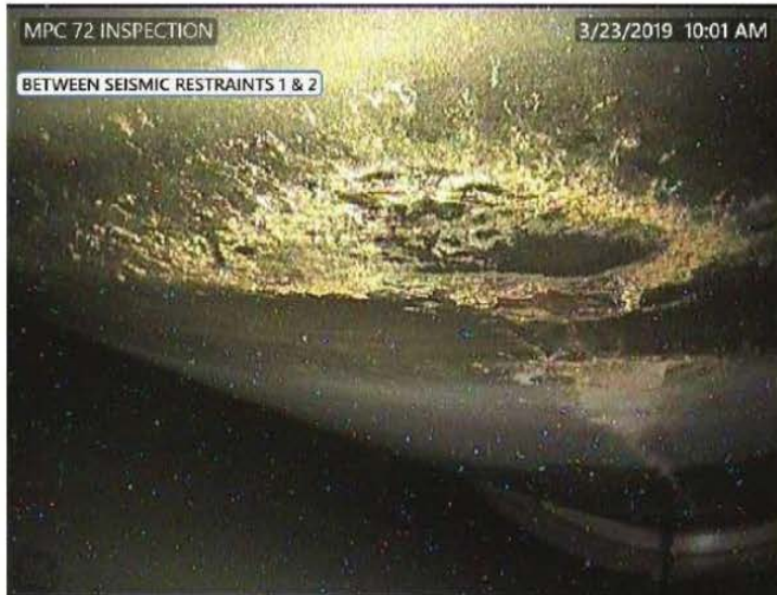
Carbon Steel Contamination within the HAZ of the MPC circumferential weld
