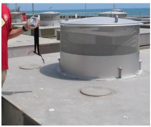
Holtec UMAX lids with large air vents. Round top has outlet air vent. Lower rectangular part of lid has inlet air vents near all corners. Radiation reading at San Onofre were 324 CPM (counts per minute) with no leaks in canister. Carbon-14 is one type of radioactivity released through the air vent. NRC only requires radiation monitoring once a quarter. No monitoring system exists to alert before leaks in canisters.
