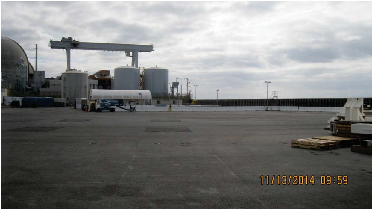
Key View 6 - View of project site looking towards Units 2 and 3.
