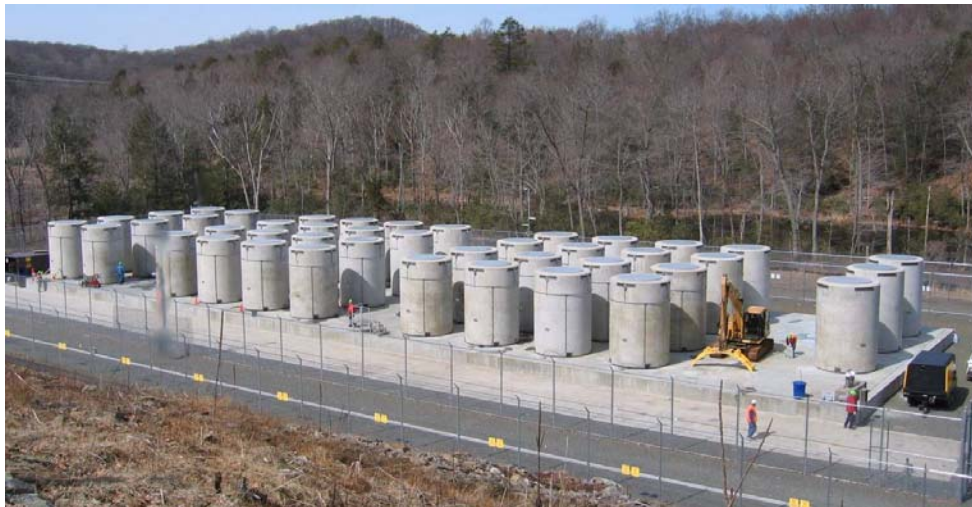
Figure 11. Independent Spent Fuel Storage Installation at Connecticut Yankee
