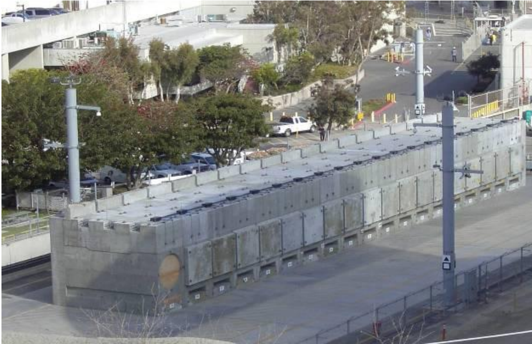
Figure 13. Transnuclear Horizontal ISFSI at San Onofre
