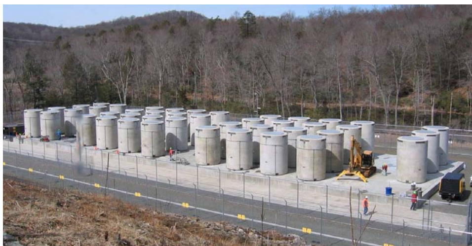
Figure 3. Independent Spent-Fuel Storage Installation
