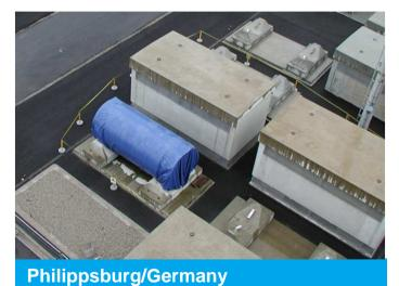
The DCI cask can be stored in a horizontal as well as in a vertical position.
